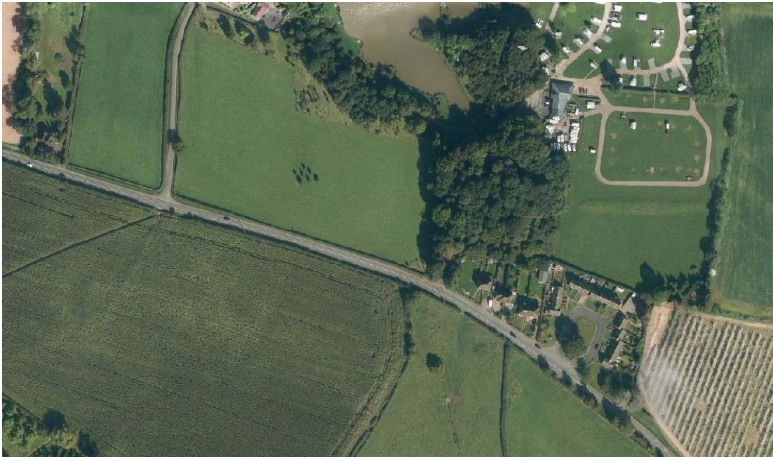
Figure 1: Recent aerial photograph of the site and context
